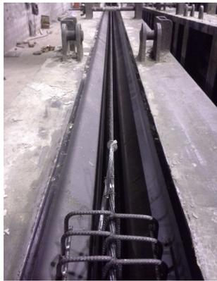
(A) Formwork with reinforcement.
